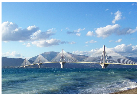
(a) The Rion-Antirion bridge, Greece
