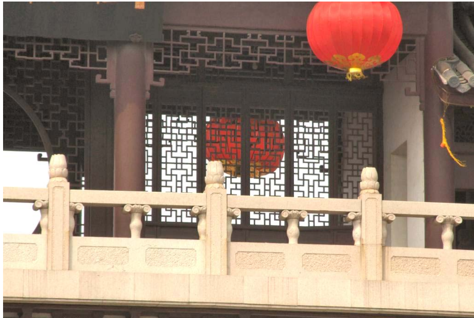
Figure 2. Lattices on the balcony of Zhouzhuang's entrance gate
